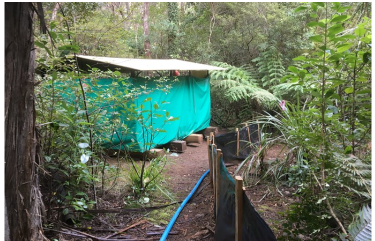
Above: A frog fence at a water pumping station. These fences are constructed from sheer polythene and remain in place until the drill site is rehabilitated.
